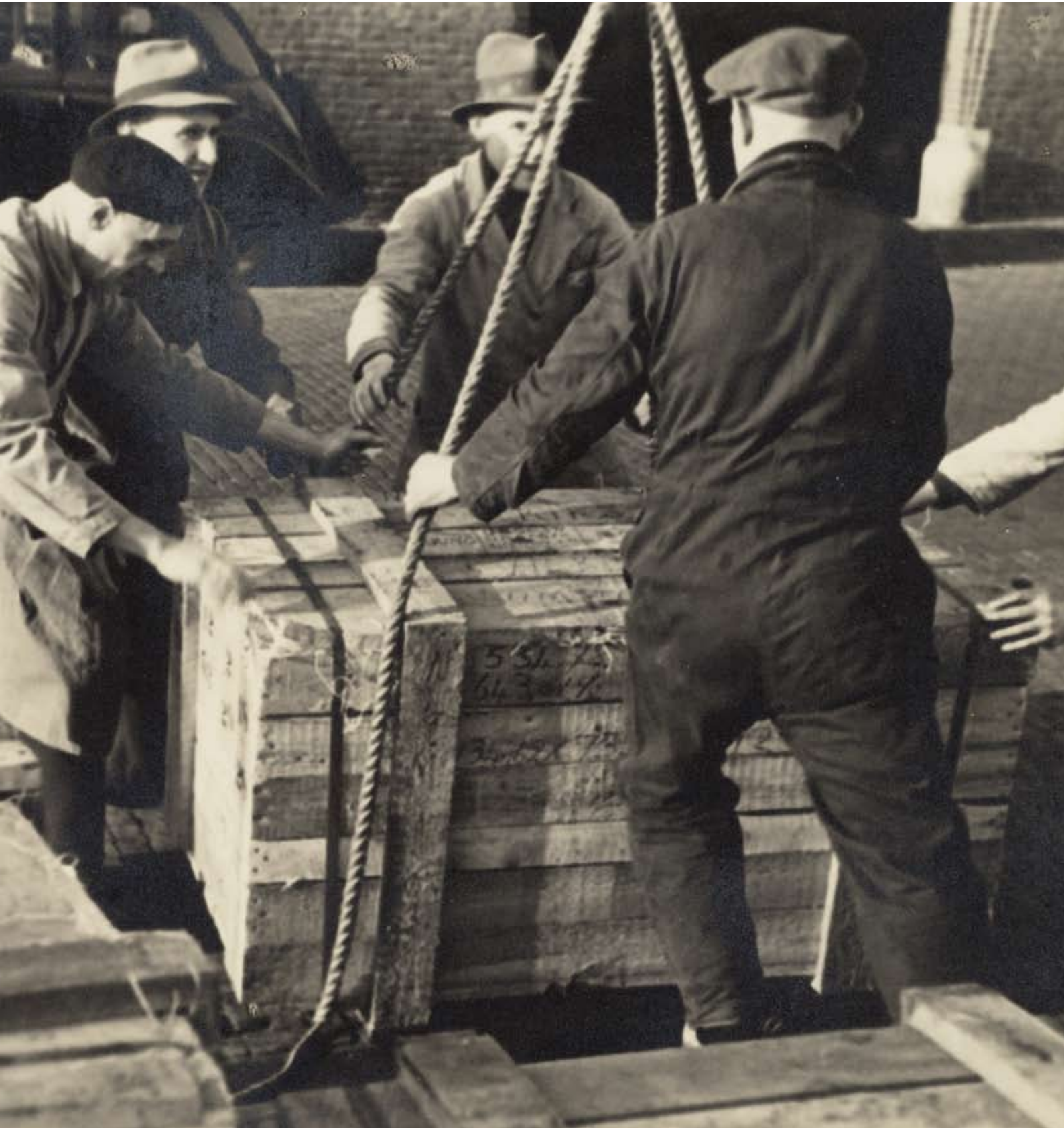
Unloading Saunders diaphragm valves at the Alkmaar warehouse
