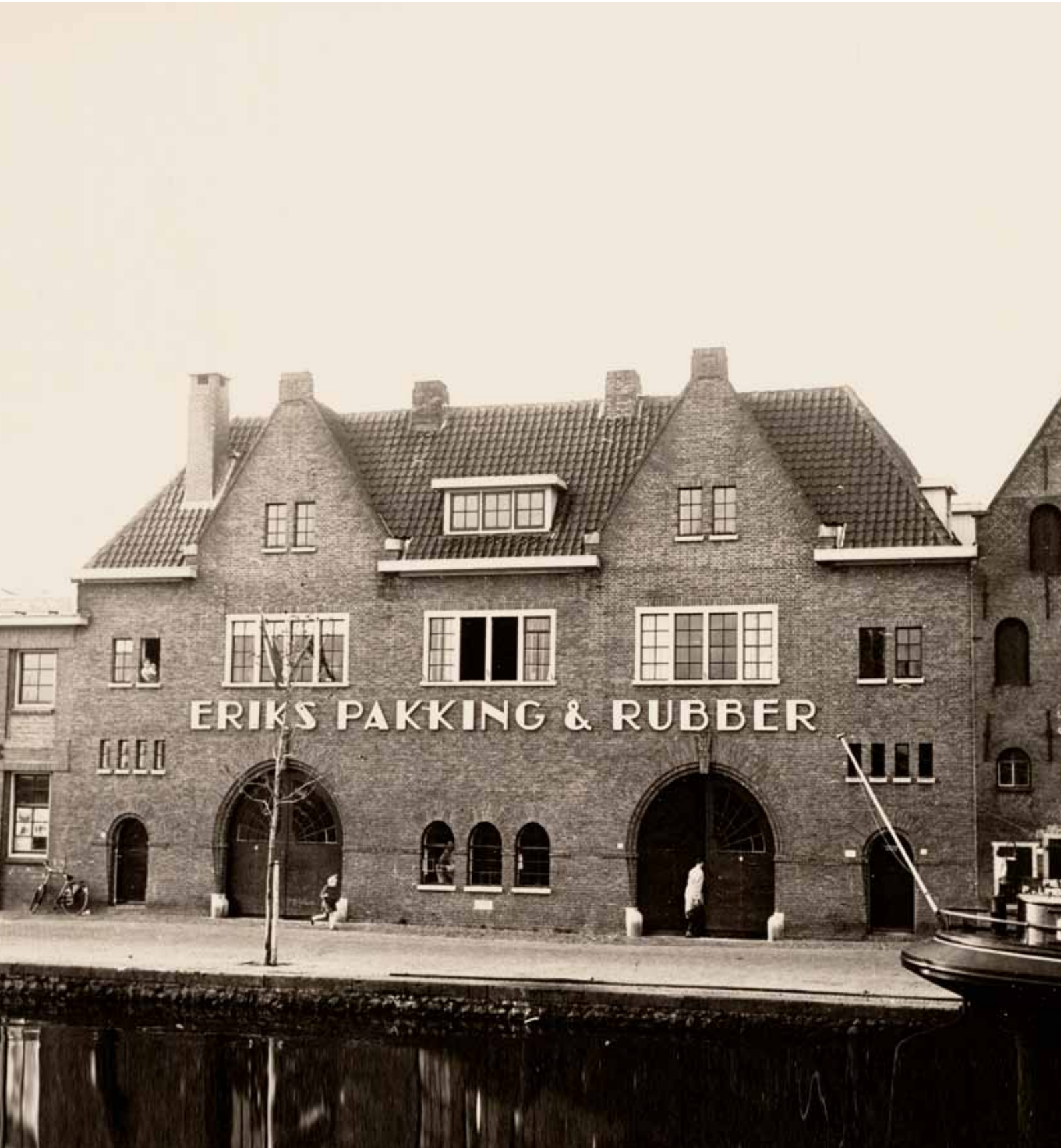
The warehouse of ERIKS Gaskets & Rubber in Alkmaar, the Netherlands.
